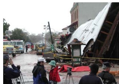
2003 San Simeon Earthquake Photo taken by Mark Wilwand
